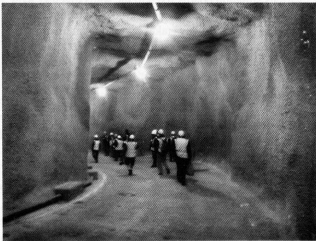
The inclined curving access tunnel that leads to the main storm-water storage cavern. The pipe on the left is used for water to clean the 'sludge' from the facility.
